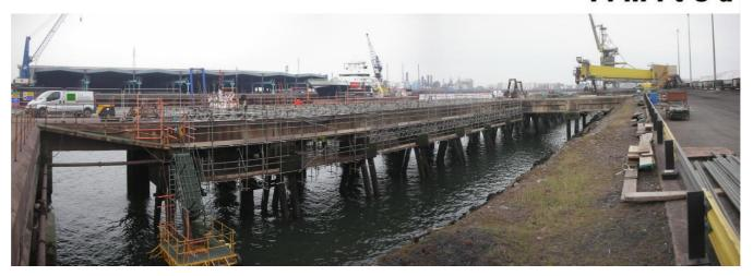
The Potash Terminal Quay is an open, reinforced concrete, type quay and is approximately 400m long. The structure enables seafaring vessels with storage capacities of some 33,000 tonnes to dock, in order to load cargo & bulk materials, before setting sail. For this reason the Quays ability to function is vital to the client.
